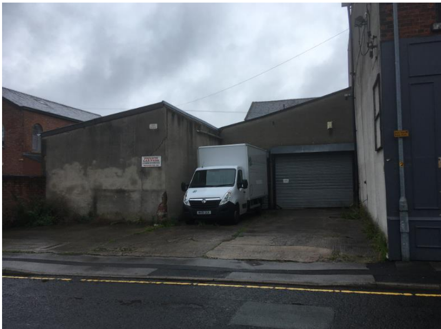
Photo 5: Lean-to to be demolished.
